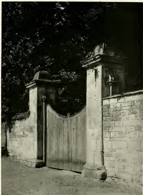
MAIN GATE IN WALL OF AN ESTATE AT BURFORD
